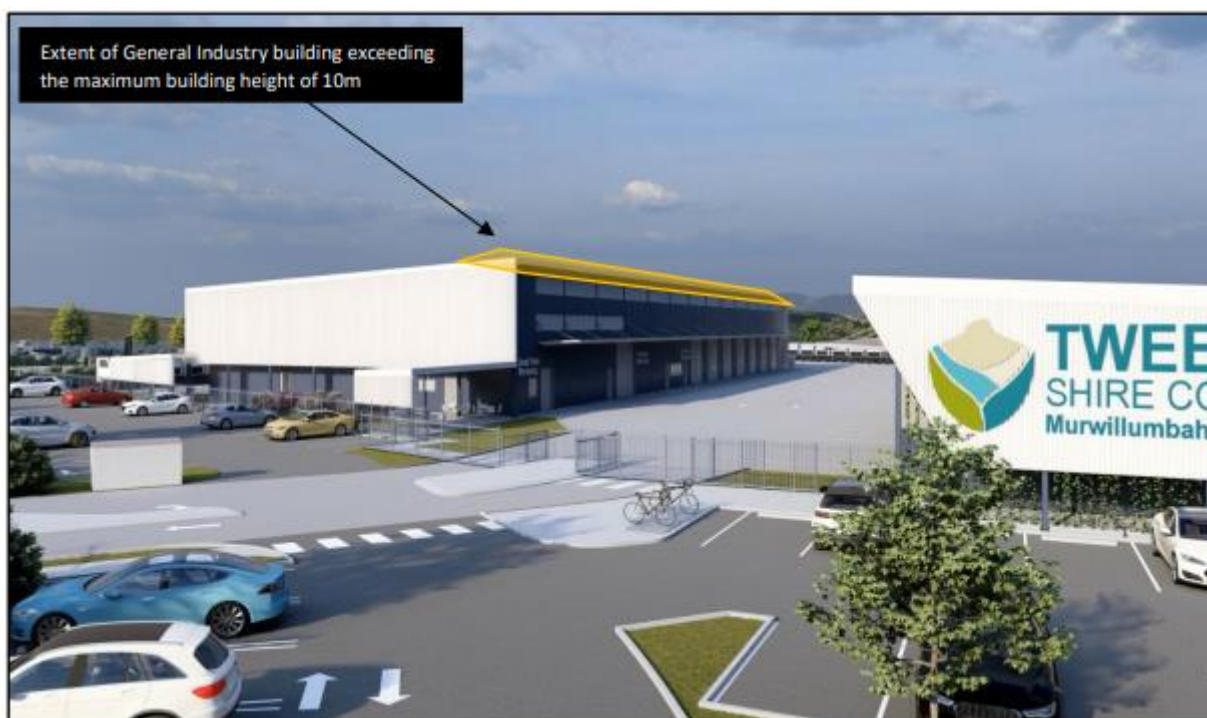
Figure 3: Render of proposed workshop building and portion exceeding the building height (Source Peddle Thorp Architecture)
